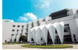
Tainan Plant (Diamond-rated Green Building)
