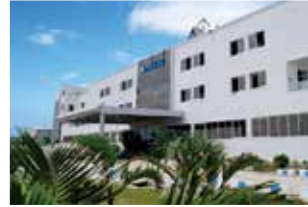
Rudrapur Plant (Green Building)
